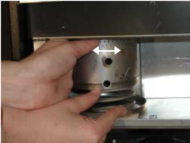
Fig. 15: Installation of the burner.
